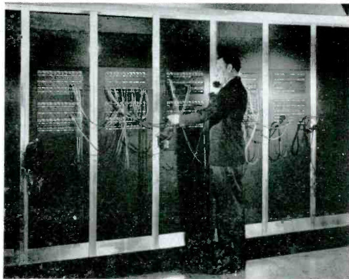
Here's Master Control Engineer Russ Hoff again. This time he's running down pops on the Red and fade-up on the Blue (we want to be impartial). "CT" has reported it as "West of Denver". Reading left to right, we see: Three remote-line termination bays, the astounded Mr. Hoff, network and special lines bay, and the outgoing lines bay.
